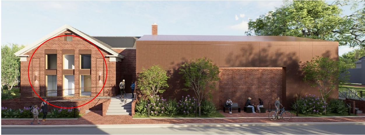
West Façade – Village Court-side
